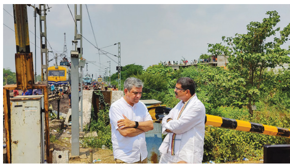
Union ministers Ashwini Vaishnaw and Dharmendra Pradhan take stock of the ongoing restoration work at the accident site in Balasore on Sunday. — PTI
