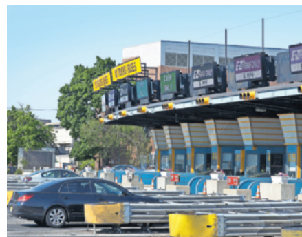
Toll lanes on major bridges on Pennsylvania interstates are being eyed as a way to fund repairs or replacements to these aging bridges with any leftover money going to pay for other transportation projects. Delaware River Port Authority
